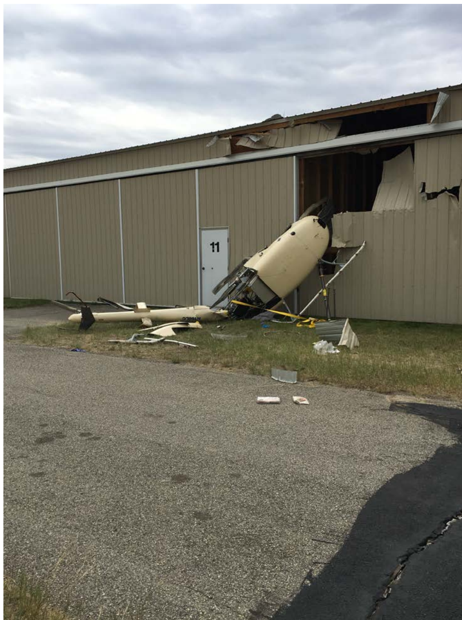
Photo 3 – view 3 of accident site
