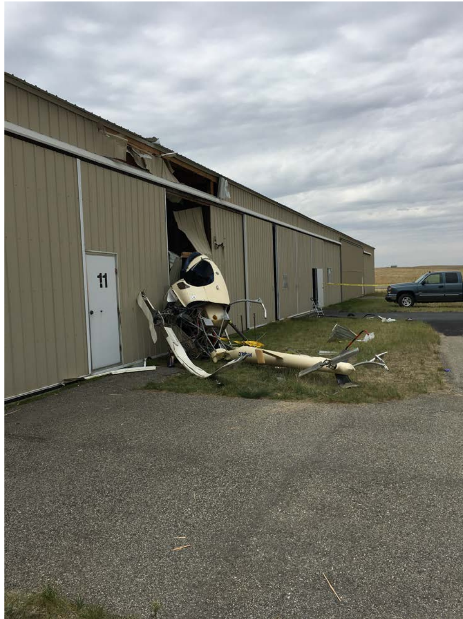
Photo 2 – view 2 of accident site
