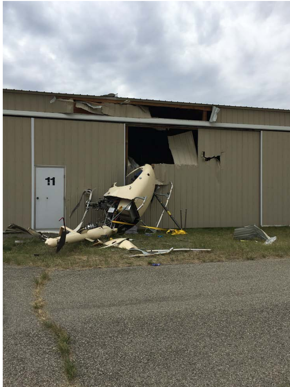
Photo 1 – view 1 of accident site
