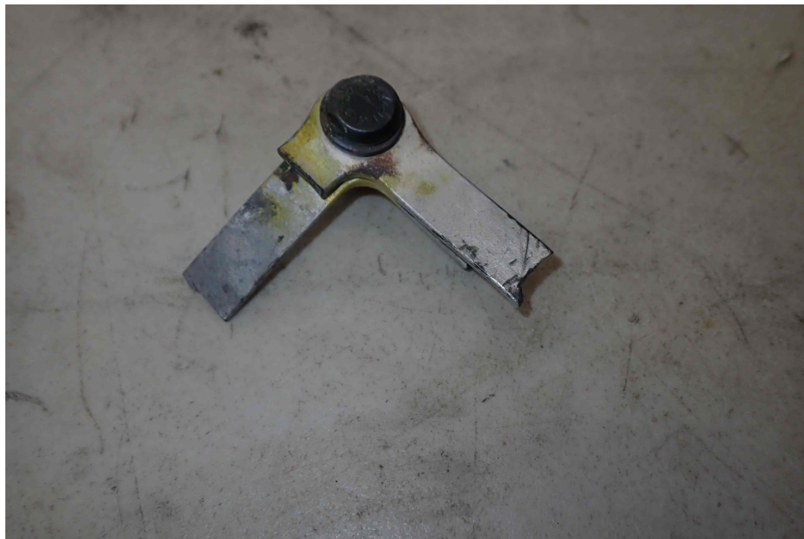
Photo 11 – Flexible Coupling Fractures
