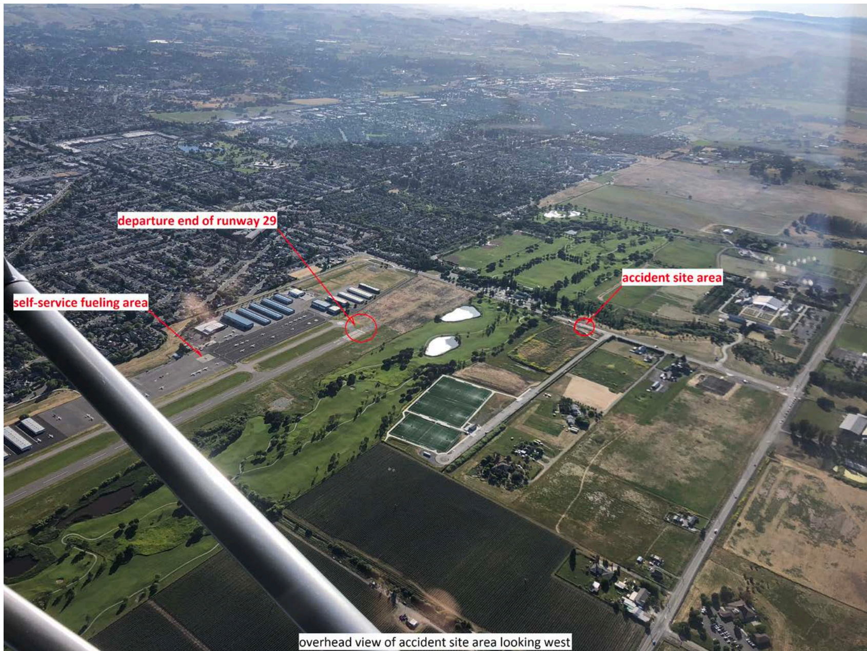
Photo 1 – overhead view of accident site area looking west
