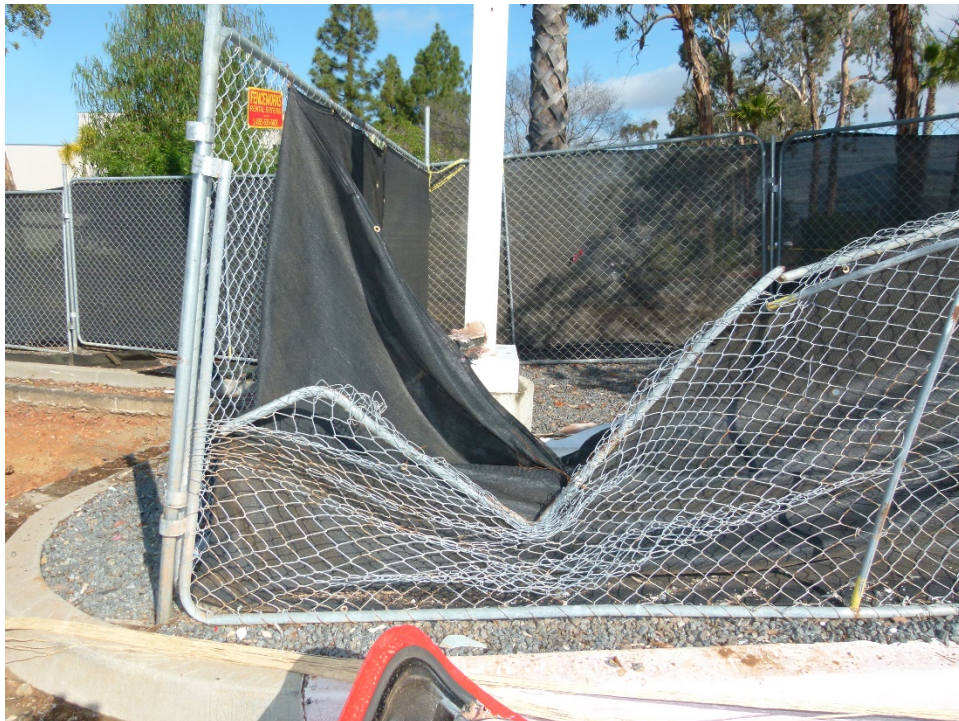
Figure 5: Damaged Fence Consistent with Right Wing Impact
