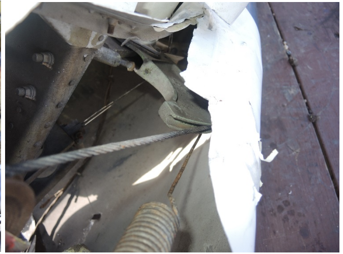
Left rudder cable on rudder horn
