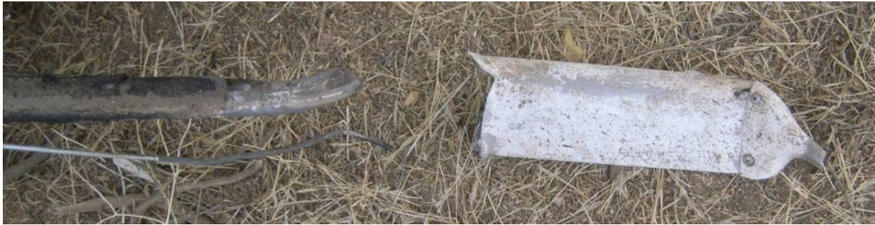
Figure 34 - Fractured End of RMLG Strut
