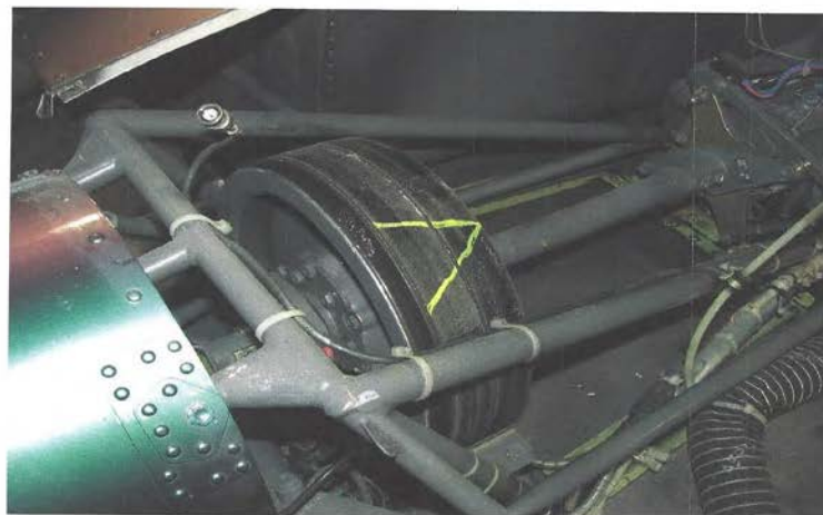
The drive belts at the upper sheave
