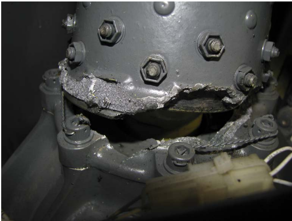
Figure 6 - photo 3 of main rotor gearbox fracture surfaces
