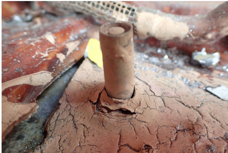
Photo 3 – Right Tank Sump Drain
