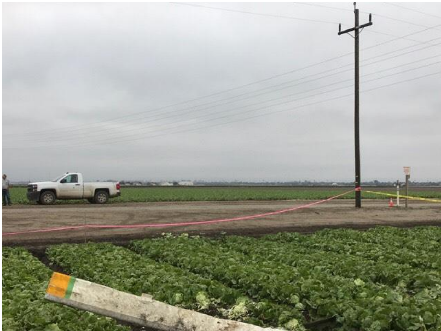
Photo 8 – Accident site, 40-ft power pole and wires.
