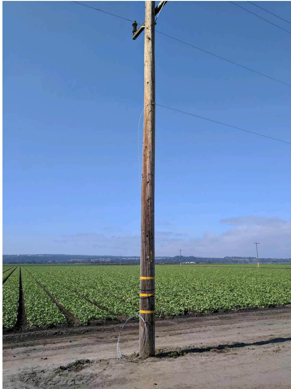
Photo 5 – Accident site, 40-ft power pole.
