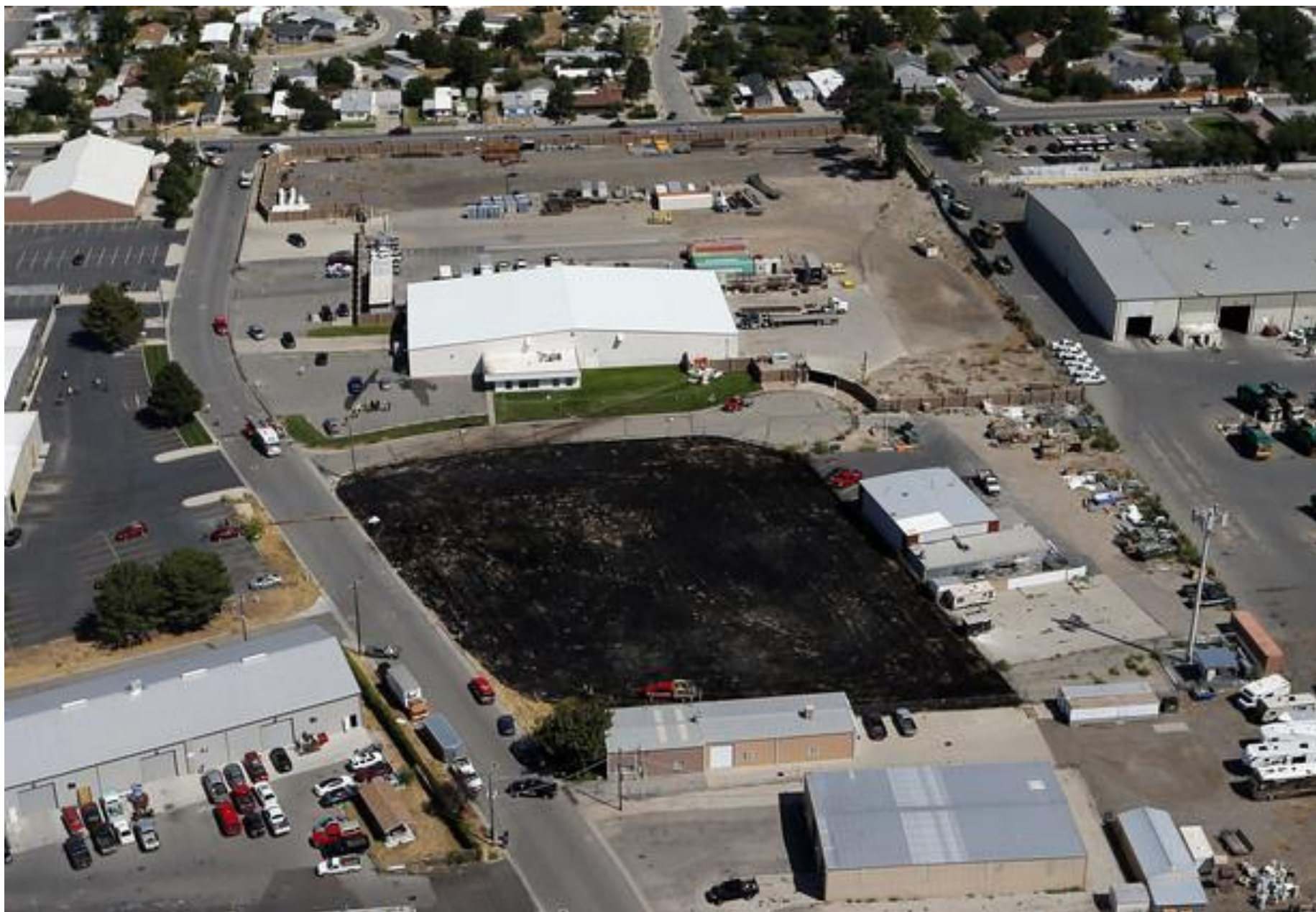
Photo 1 – Aerial view of the accident site.
