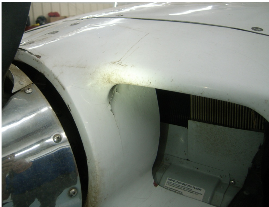
Figure 6 - Trace Oil Residue on Inlet
