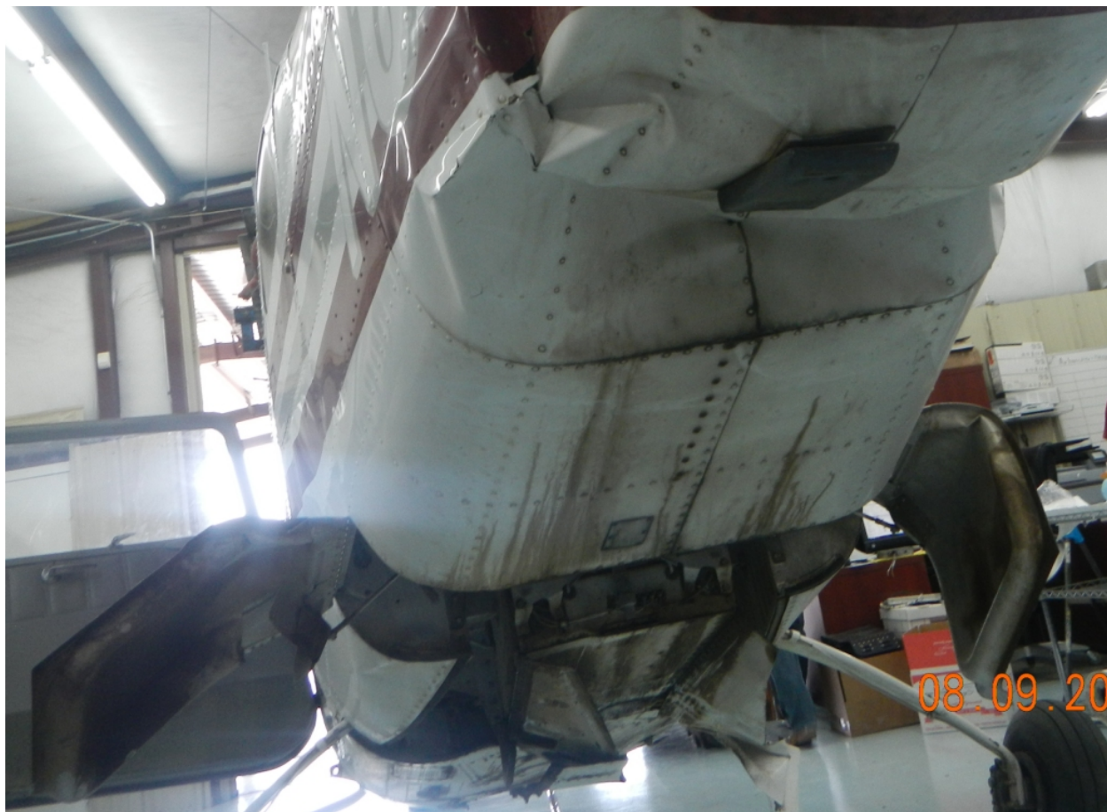
Figure 3 - Underside (view forward)
