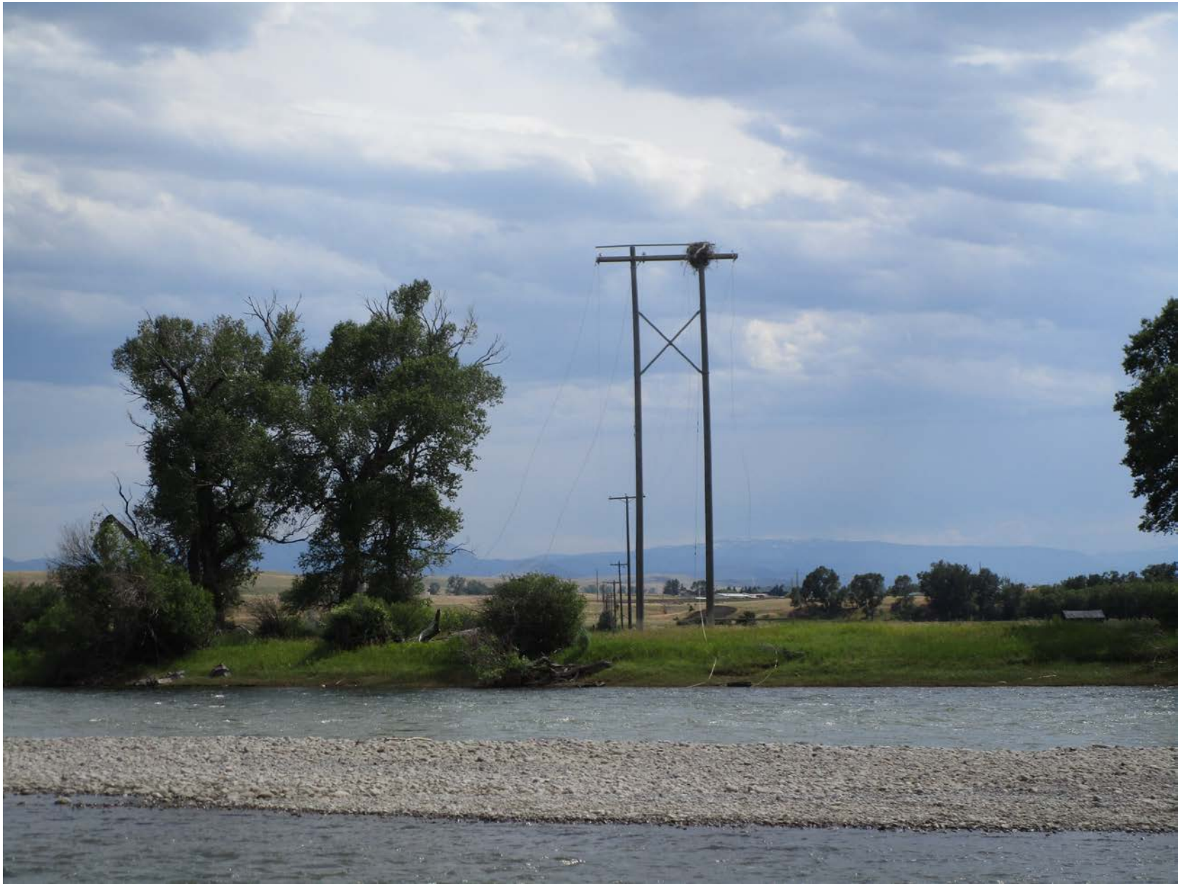
Photo 4 – View of Downed Powerlines from Water (Courtesy of Federal Aviation Administration)
