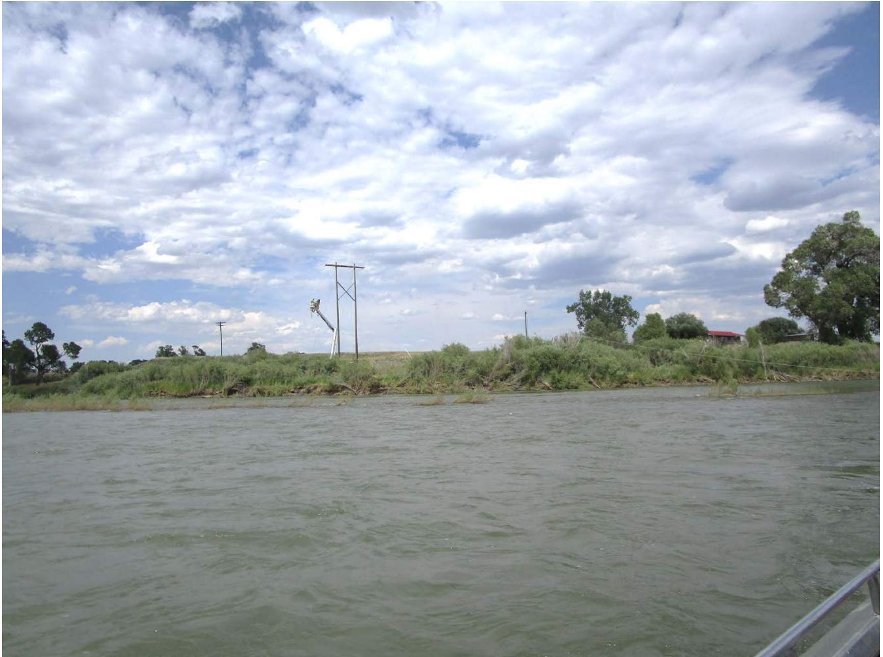
Photo 1 – View of Downed Power Lines (Courtesy of Federal Aviation Administration)
