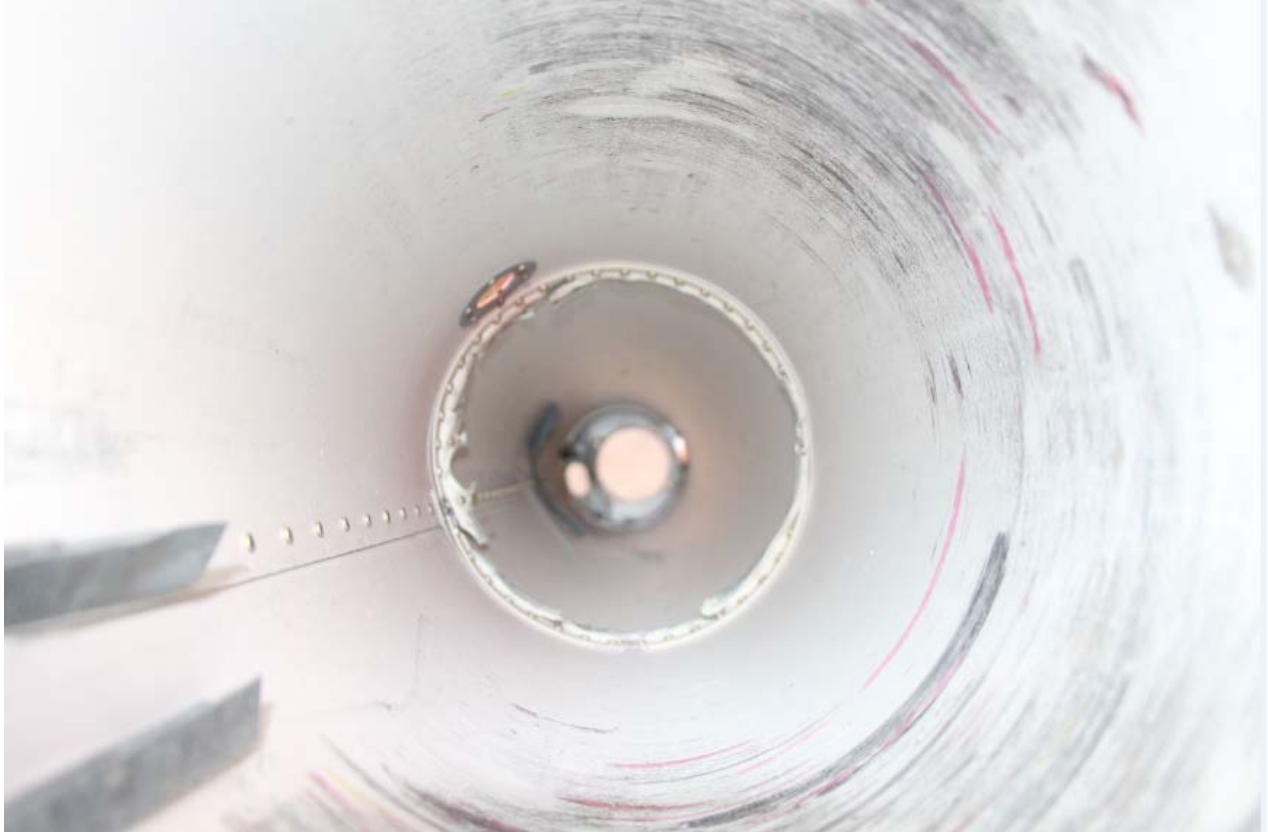
Figure 5 – Inside Diameter of Tailcone, No. 7 Bulkhead
