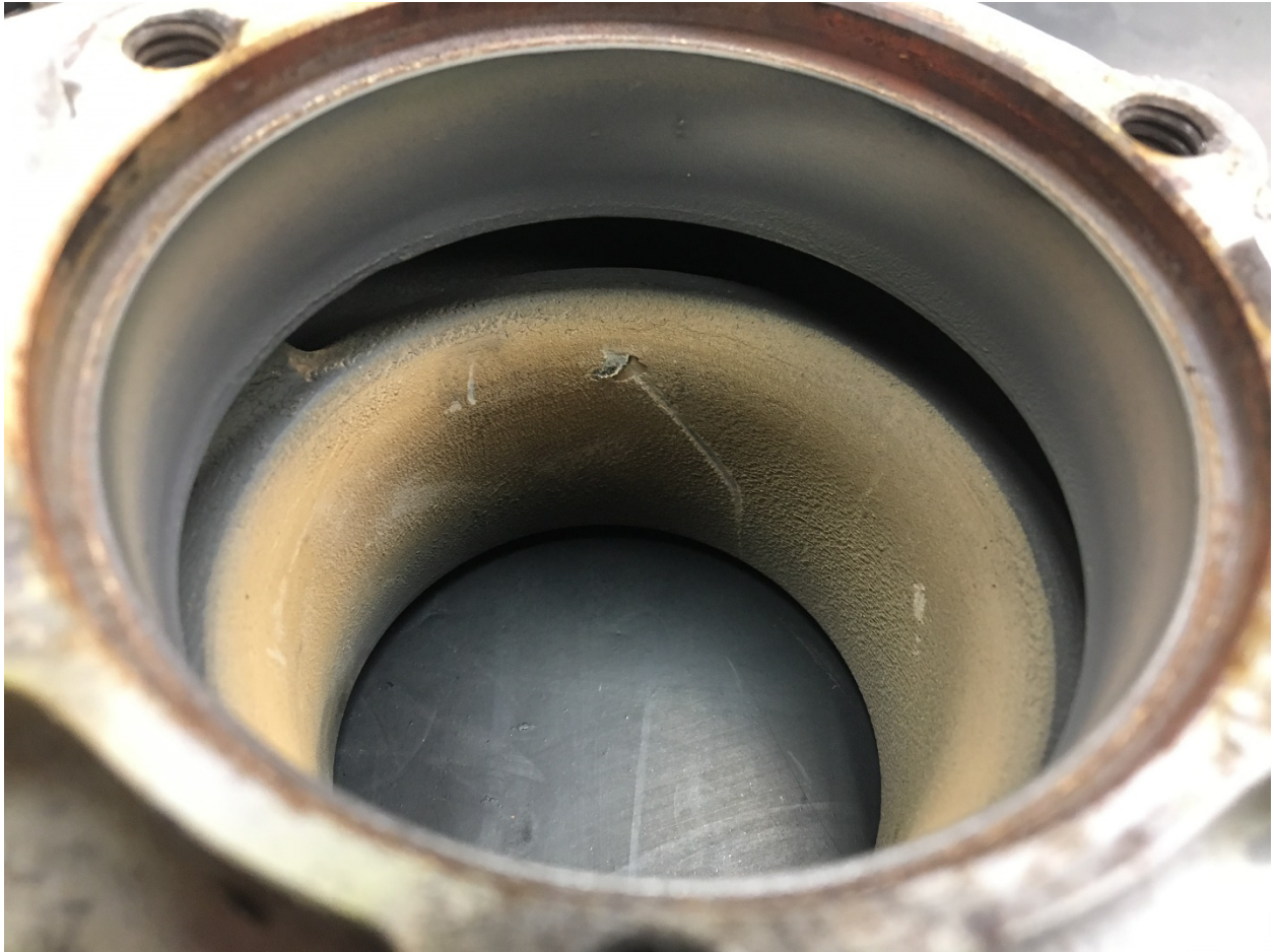
Figure 12 Turbine Housing with Witness Mark
