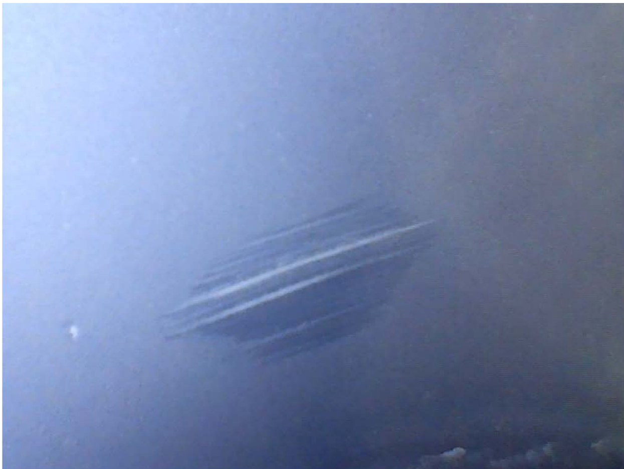
Figure 16 Scrape Mark 4 Inside Right Exhaust
