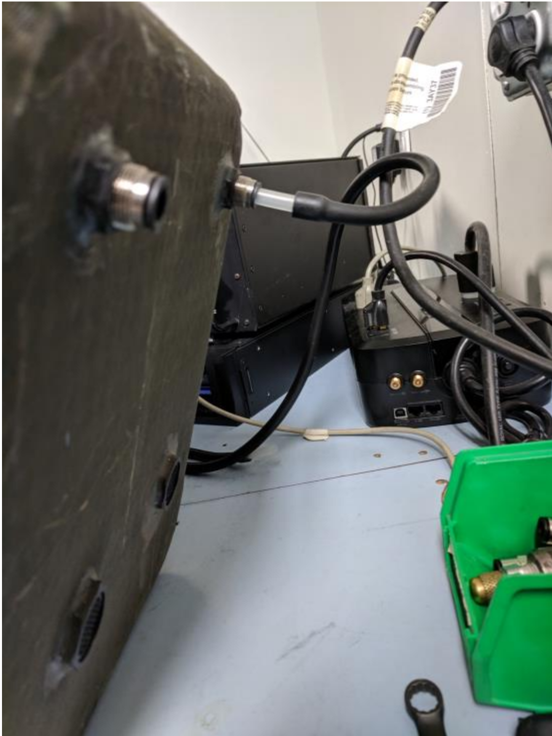
Figure 10 – Full system leak test on second static port
