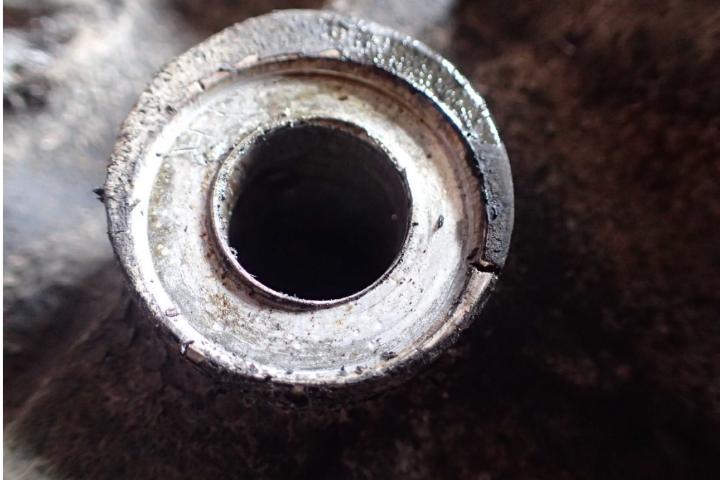
Photo 13 – Forward Carry-Through Bolt Hole
