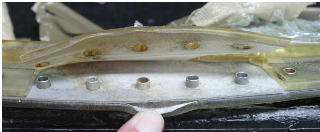
Figure 6 – Disassembled area of lower flange on left windshield
