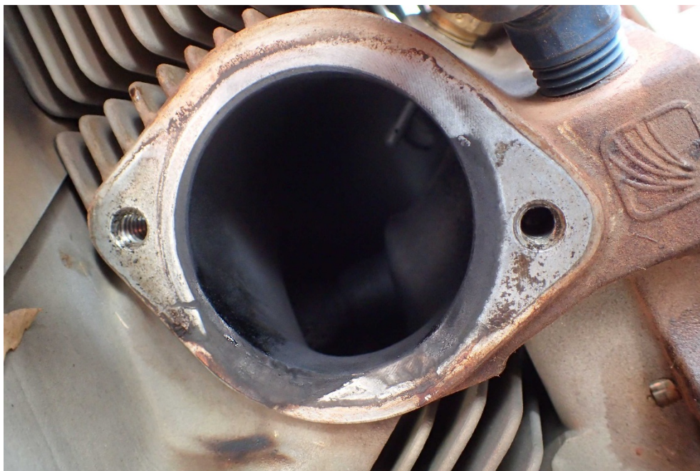
Photo 6 - Number 3 Intake Cylinder Head Flange
