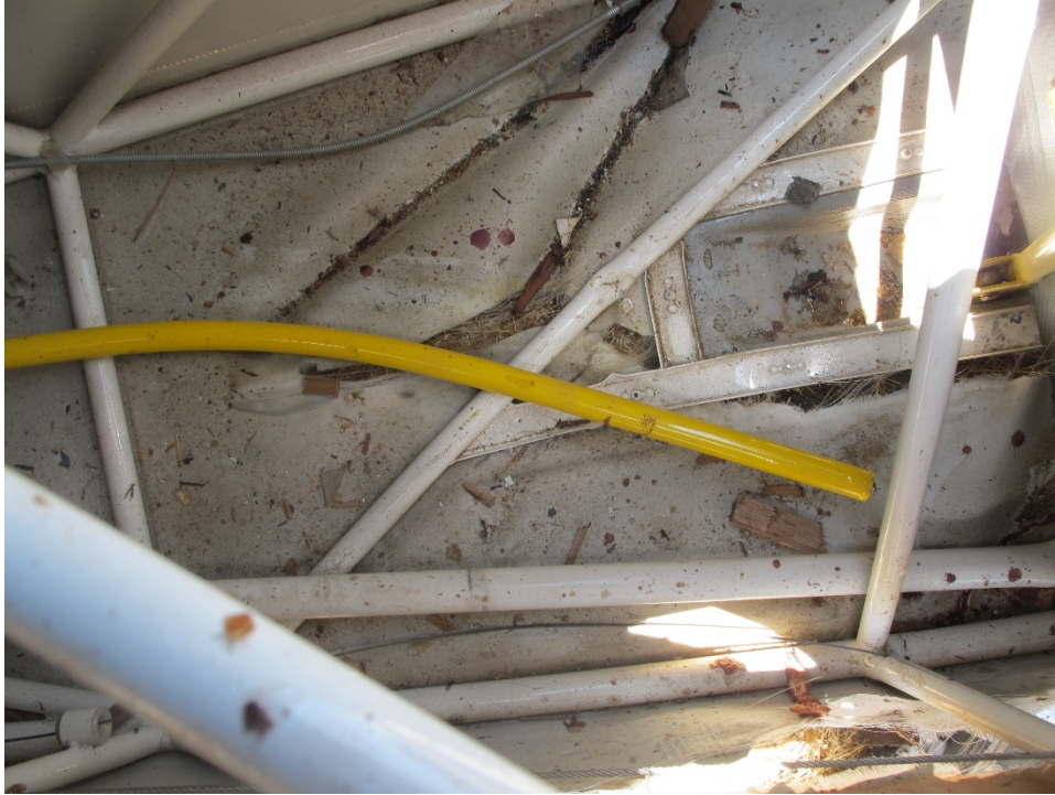
Figure 7: Fractured and Bent Elevator Control
