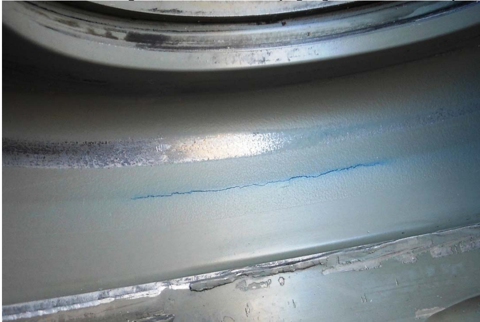
Photo #22 – Right aft hub half crack (highlighted with blue ink)
