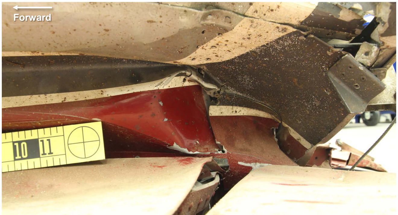
Figure 26 – Closer view of the dent in the underside of the horizontal stabilizer, showing the location where organic material was extracted.
