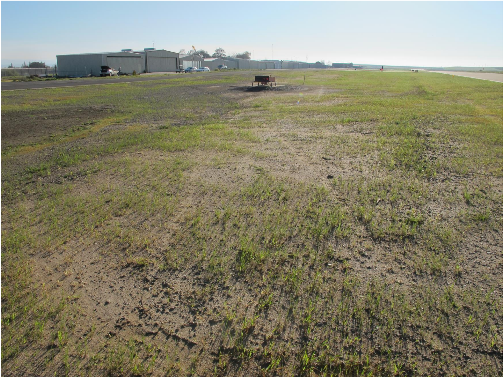
Photo 4 – Accident Site, Runway Safety Area
