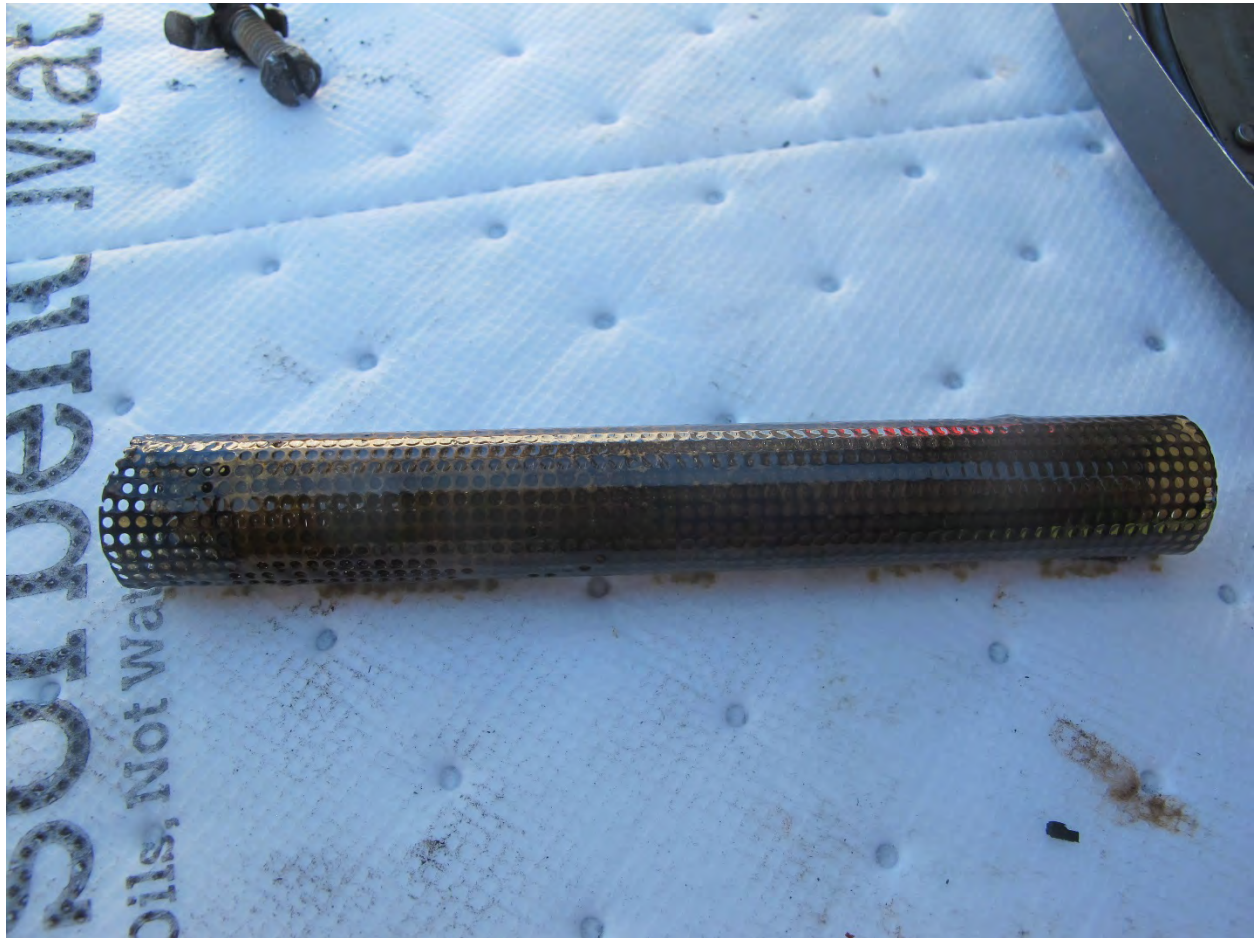
Photo 17 Oil Suction Screen
