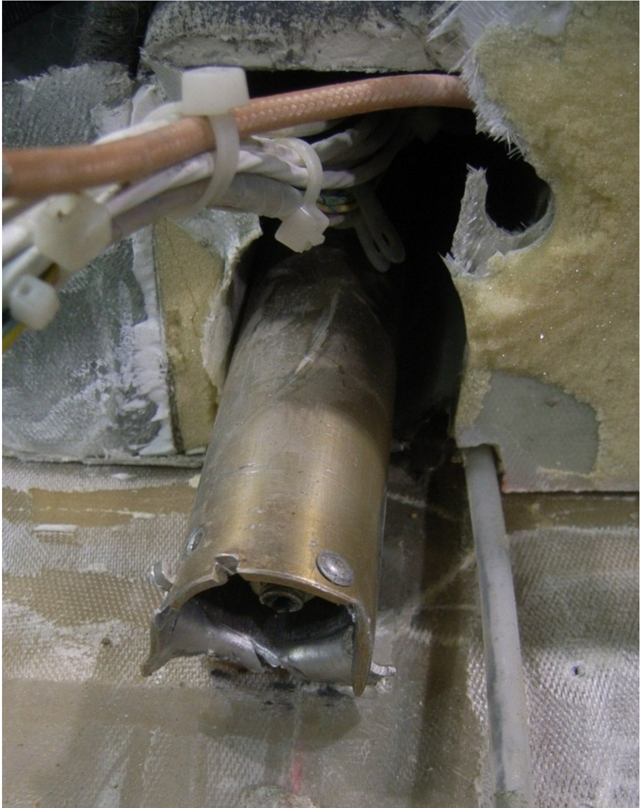
Figure 17 - Fractured Elevator Control Rod
