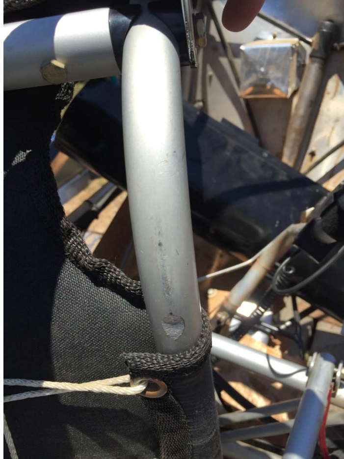
Photo 4: Wear mark on the seat frame.
