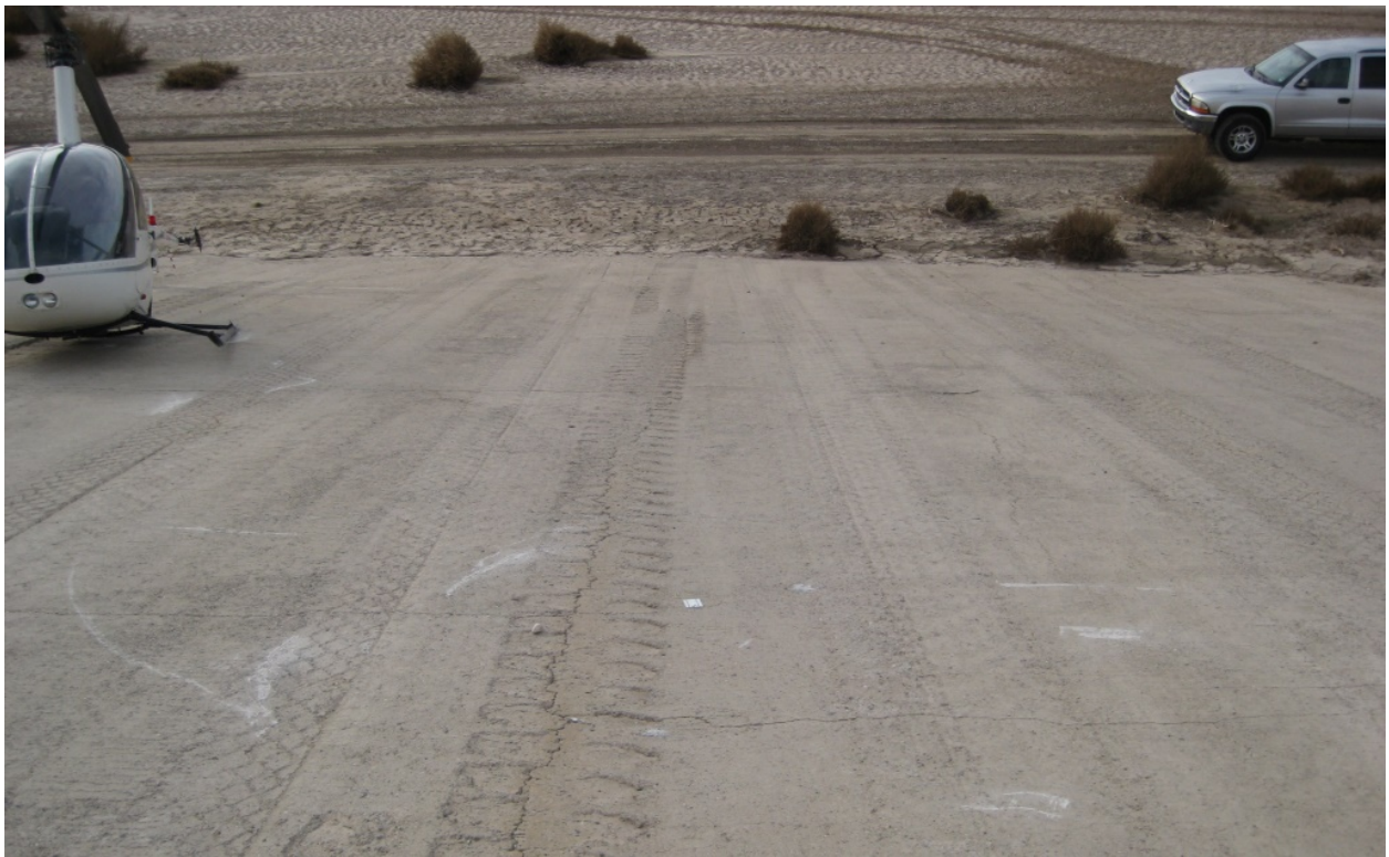
Figure 3 - Scrape Marks on Levee
