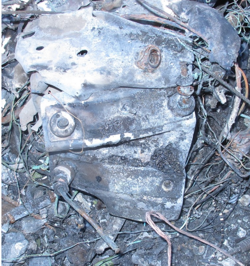
Figure 39 - Engine Control Sub-Panel
