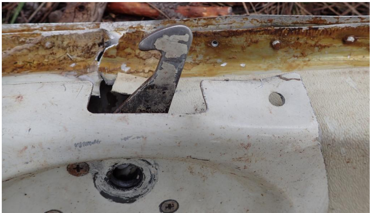
Figure 53 - Starboard Entry Door Upper Latch
