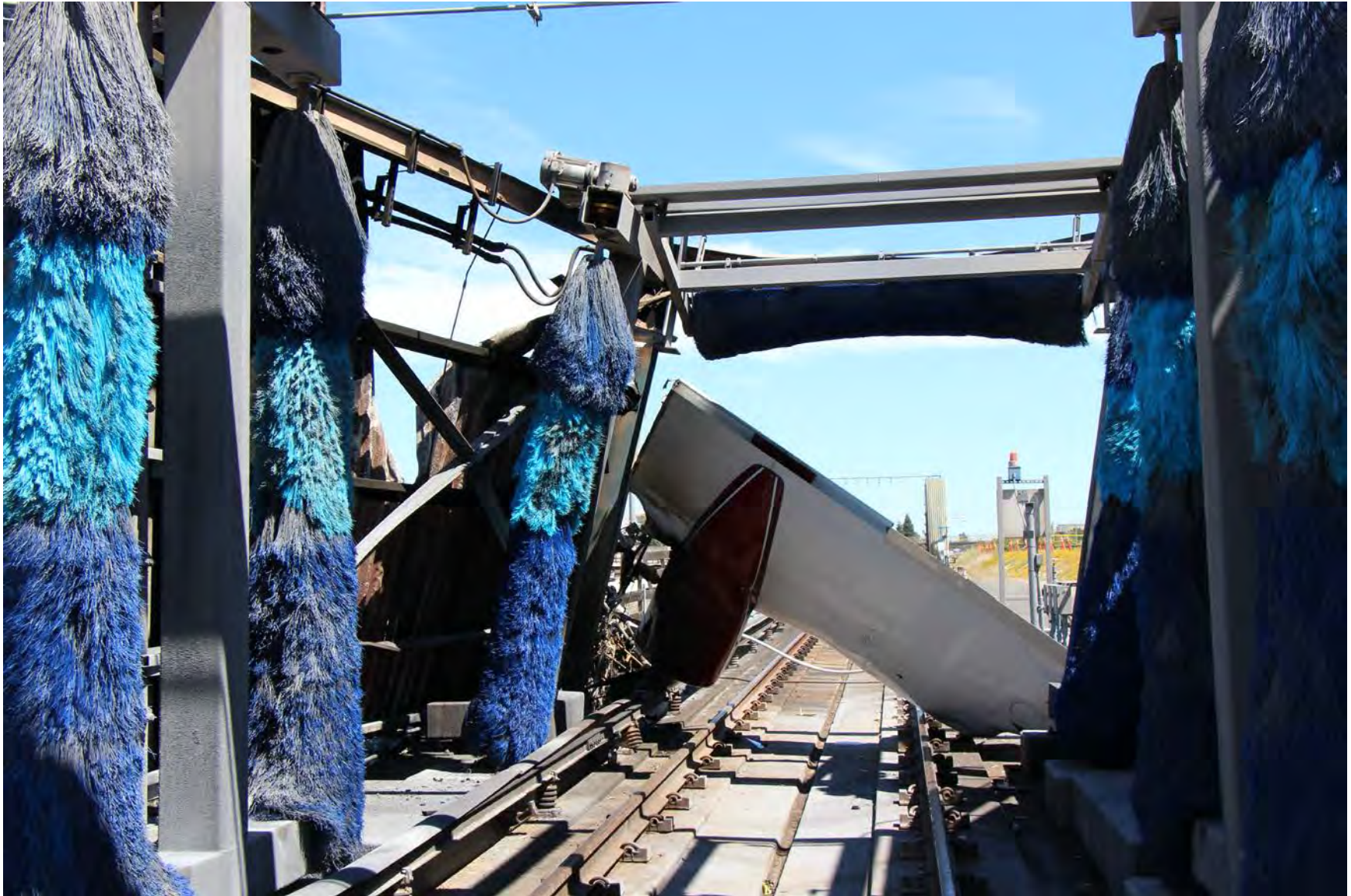
Photo 2 – View to Southeast Through Railroad Car Wash Building of Left Wing
