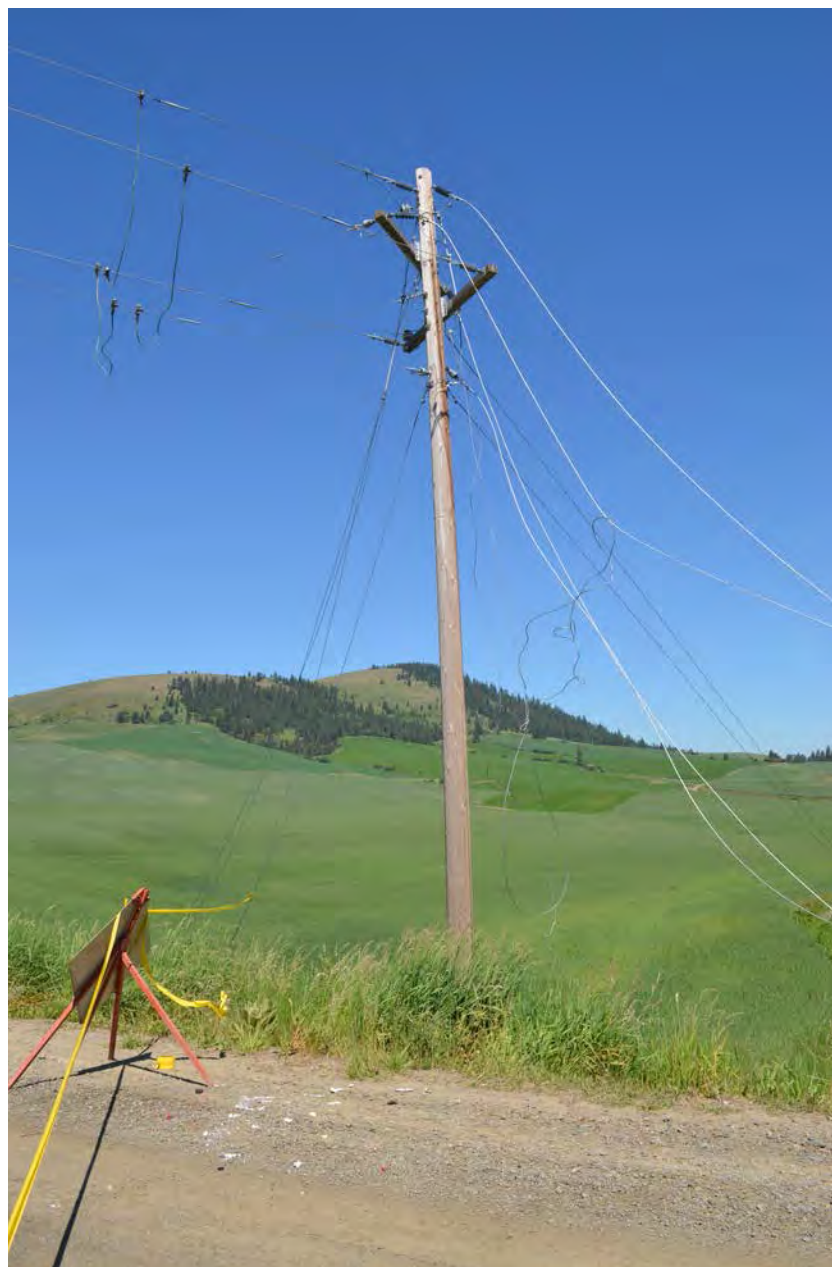
Photo 2 – view of utility pole powerlines and support guy wires
