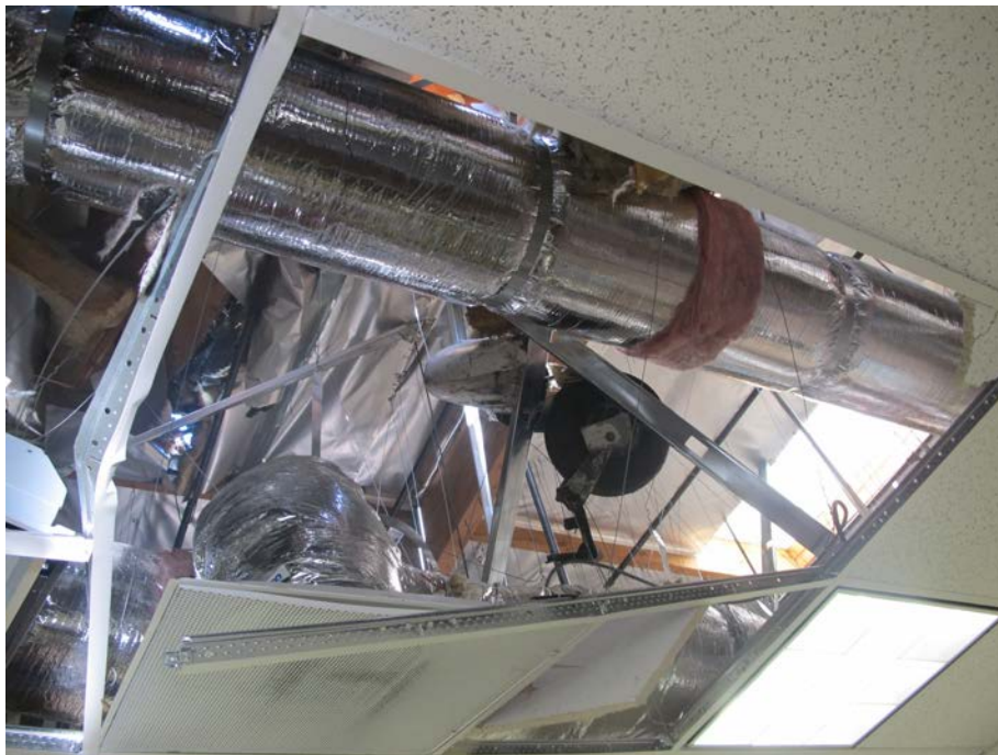
Figure 5 - separated nose wheel in ceiling of building
