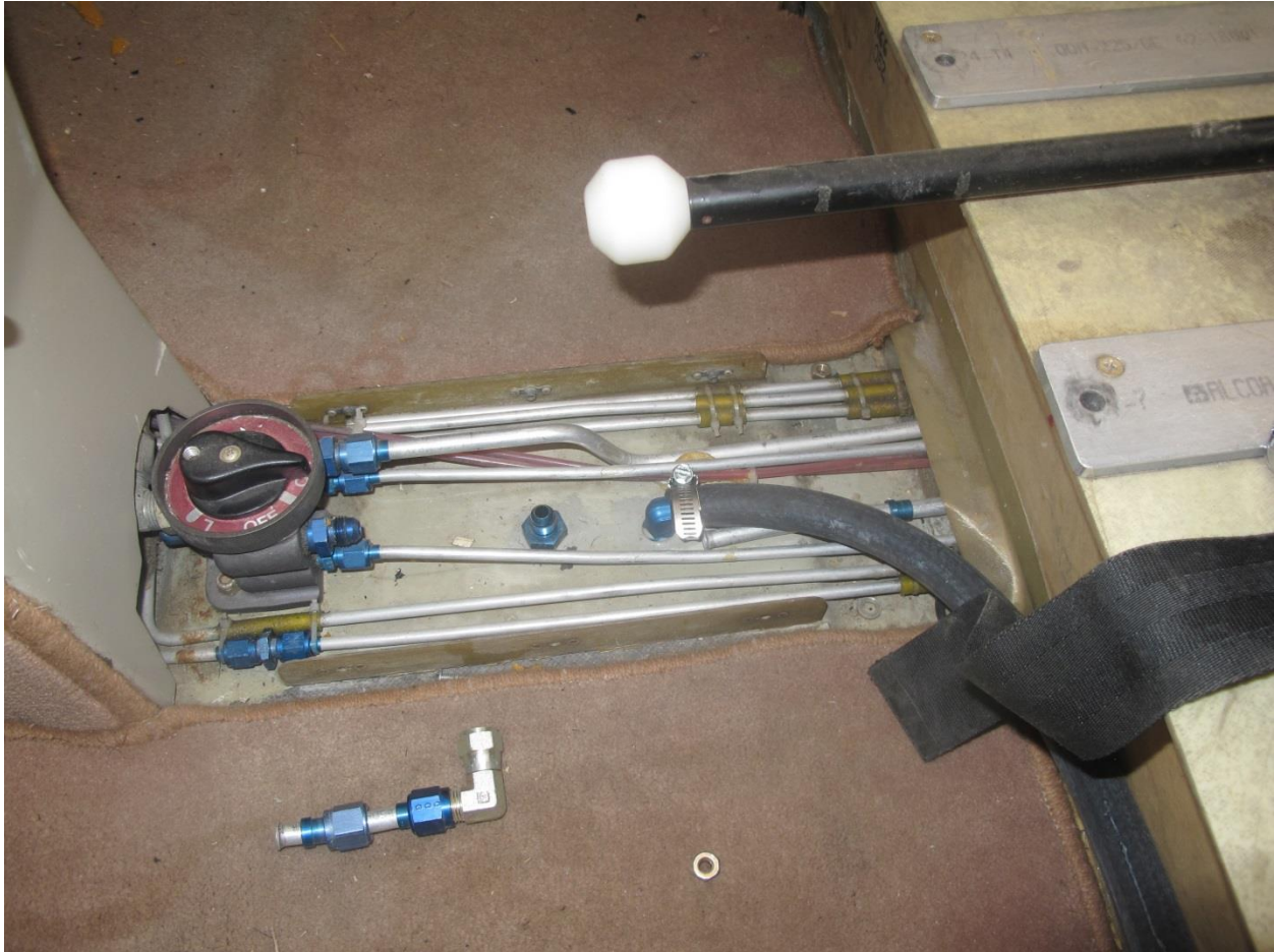
Photo 10 Fuel Lines Plumbed to Attempt Fuel Measurement
