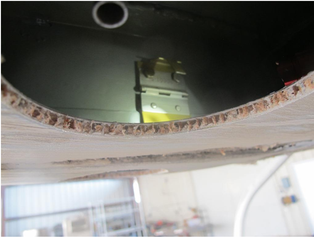
Photo 16 Flapper Valve Closed Position
