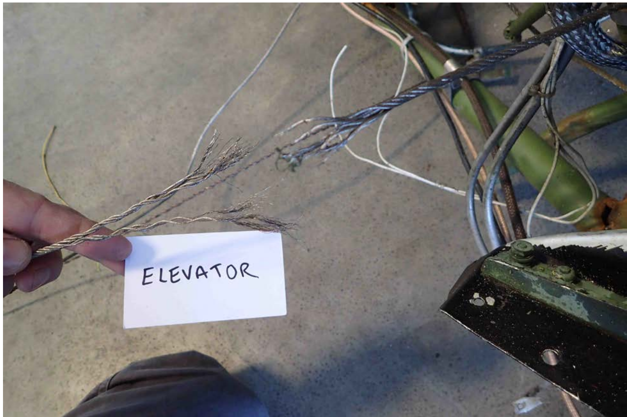
Photo 39 – Lower Elevator Control Cable
