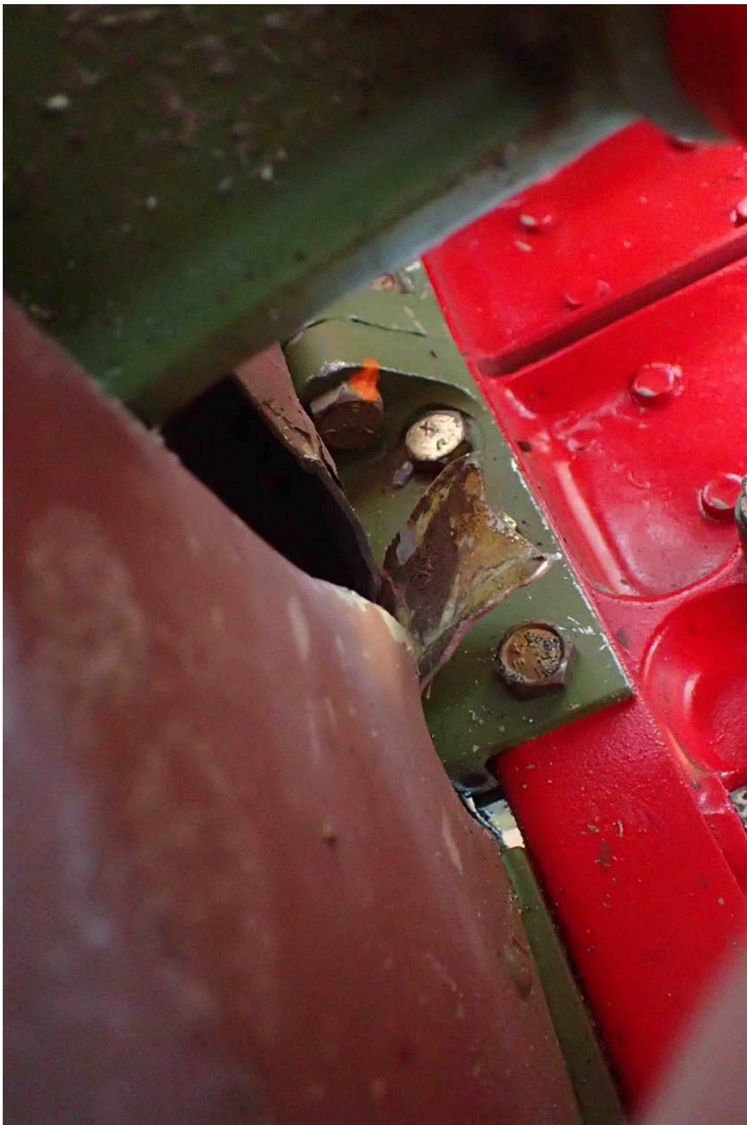
Photo 38 – Horizontal Stabilizer Deck
