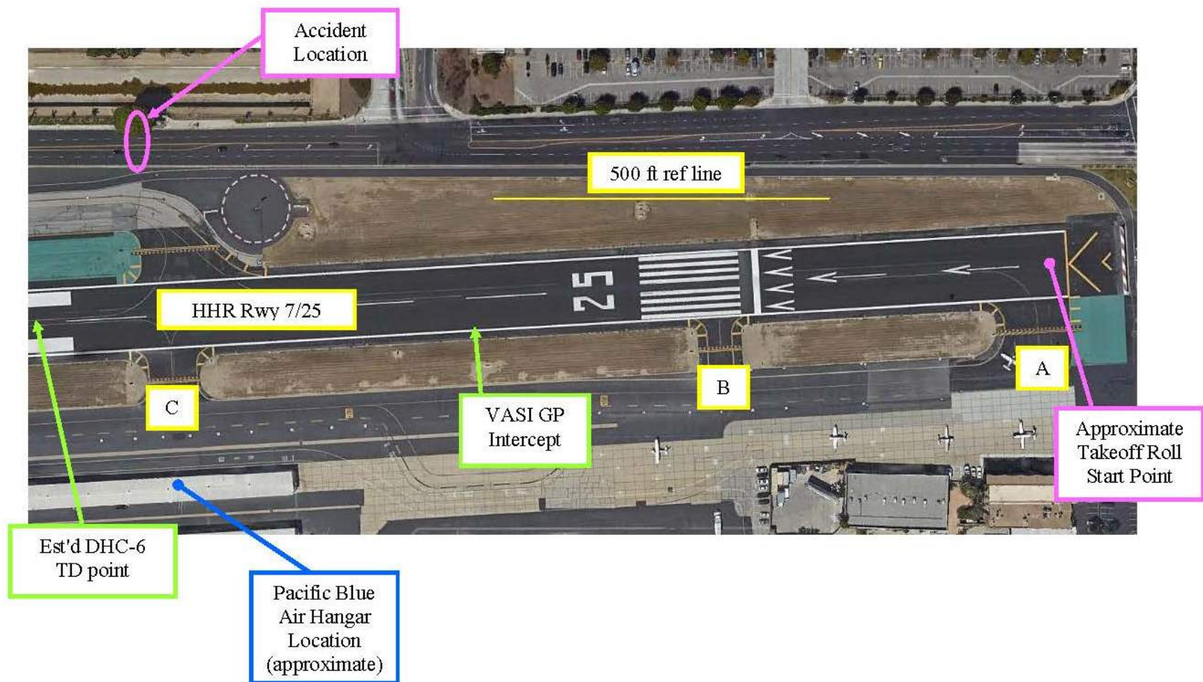
Figure 1 – Overview of HHR East End (Taxiways A, B, & C, plus other features, noted)
