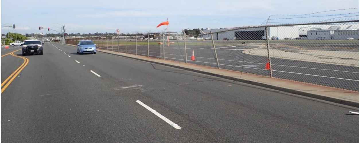
Figure 4 - Fence Damage and Ground Scar (looking east)
