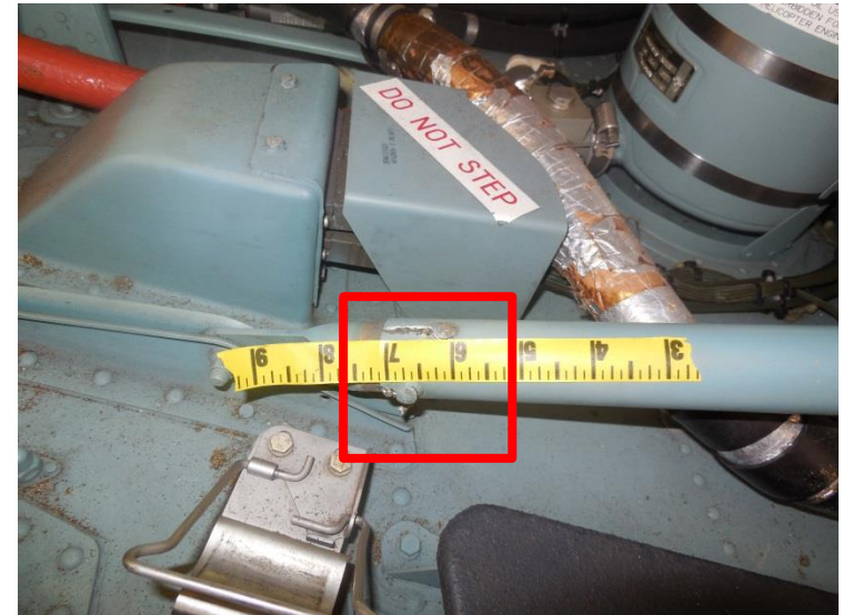
Right inclined rod lower junction
