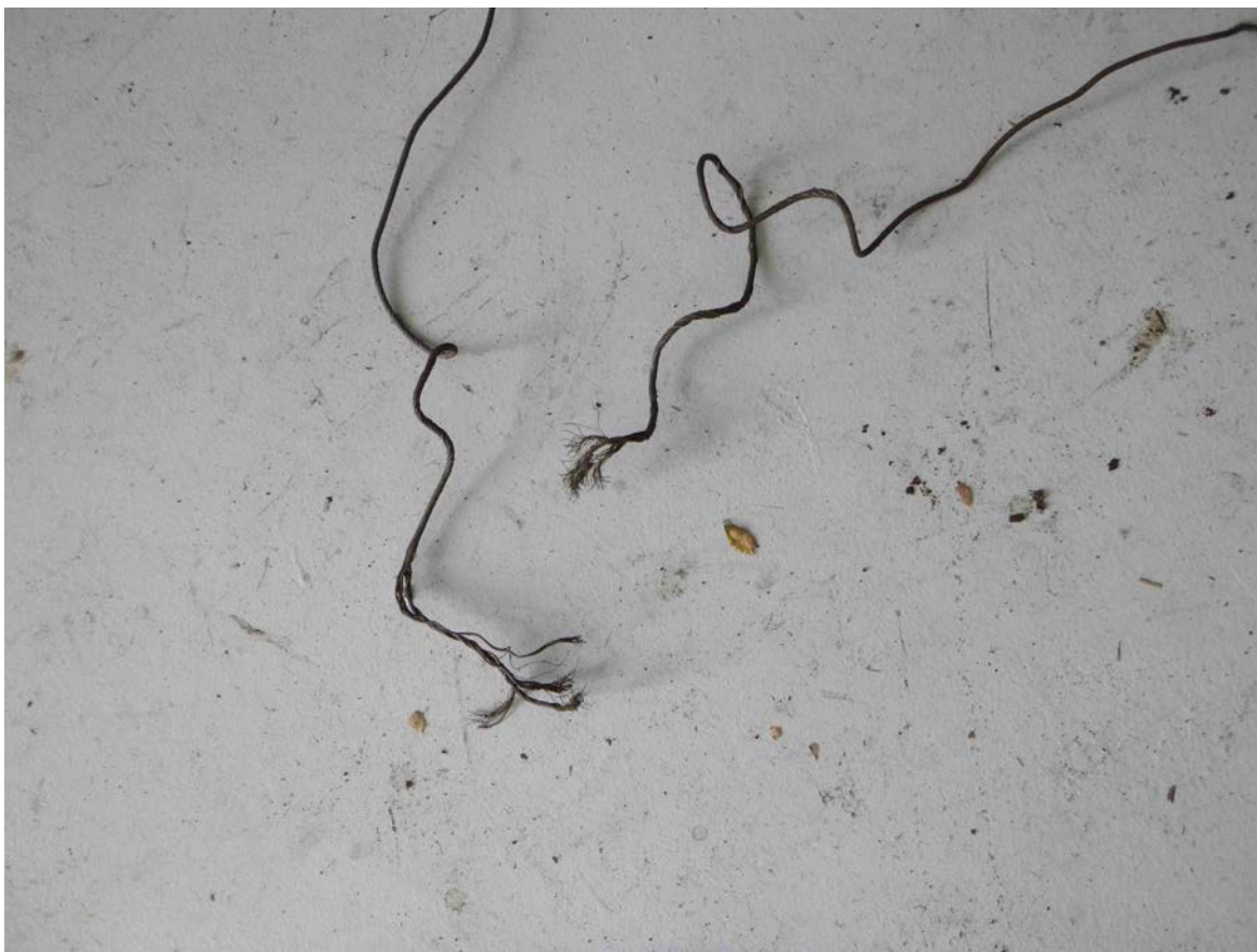
Photo 22 – Typical Cable Separation
