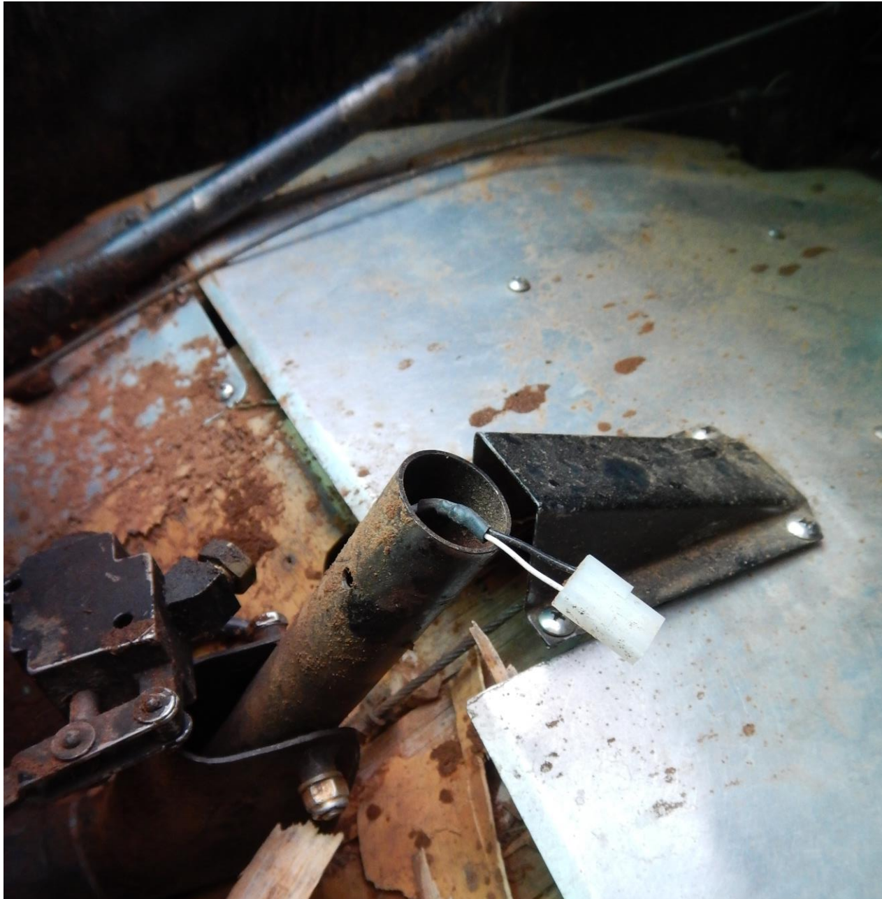
Photo 3 – The Stub and Hole for Through Bolt
