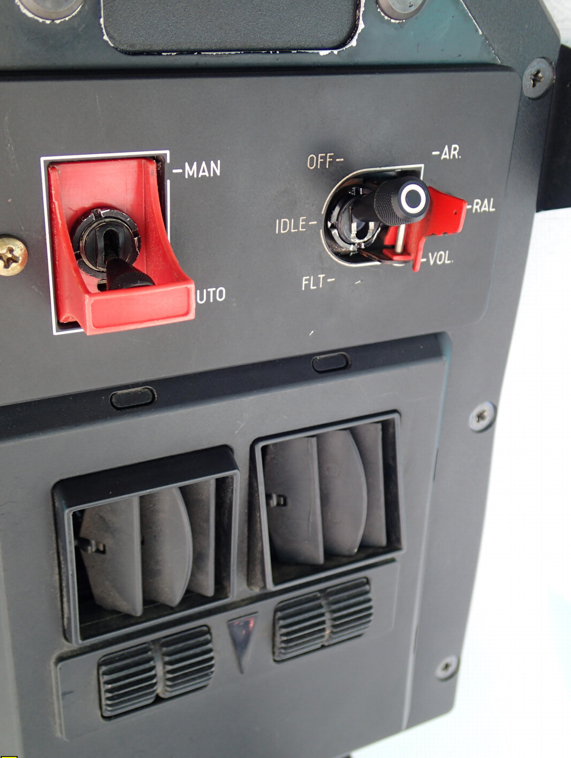
Photo 1 – Overhead Auto to Manual Switch
