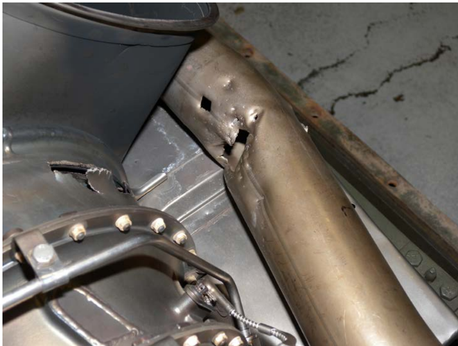
Figure 13 – Detail of Compressor Discharge Tube Damage - Inside
