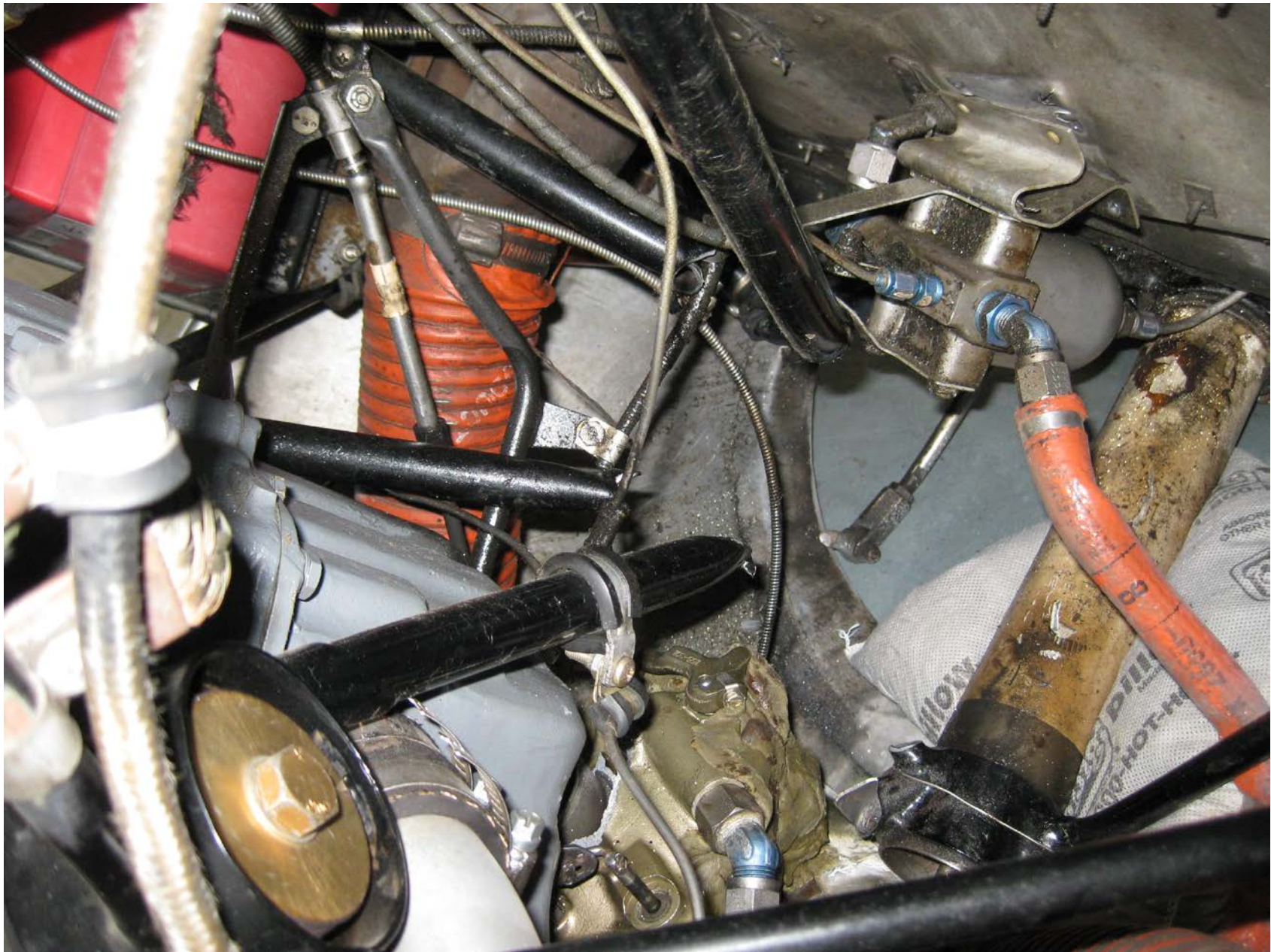
Photo – View of damaged engine mount and truss (courtesy of the FAA)
