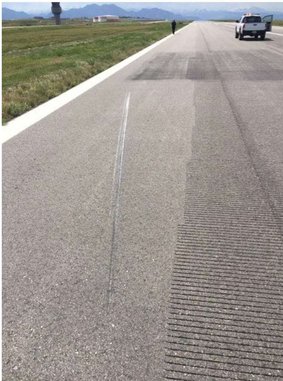
Photo 1 – View of white runway scrape marking (Photo courtesy of airport operations)
