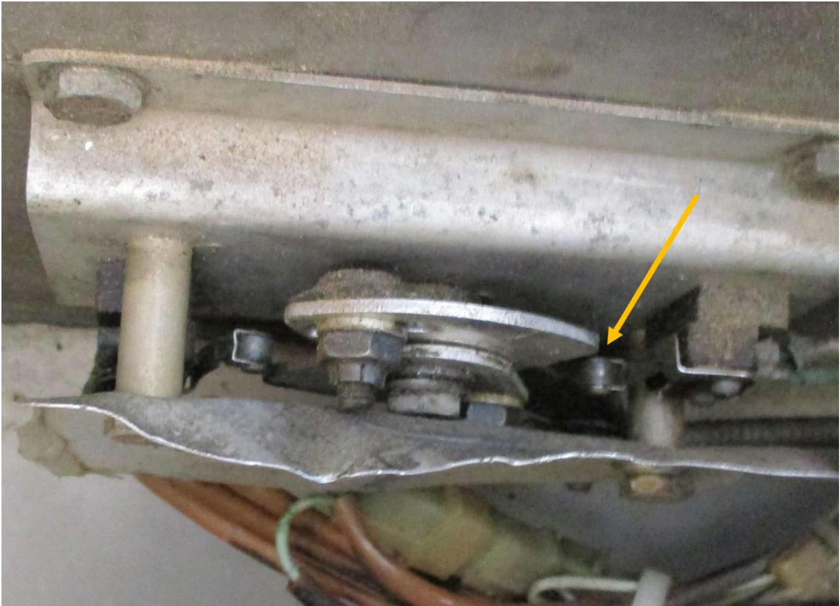
Photo 3 – View of gear warning microswitch at throttle idle position with visible gap (Photo courtesy of the FAA)
