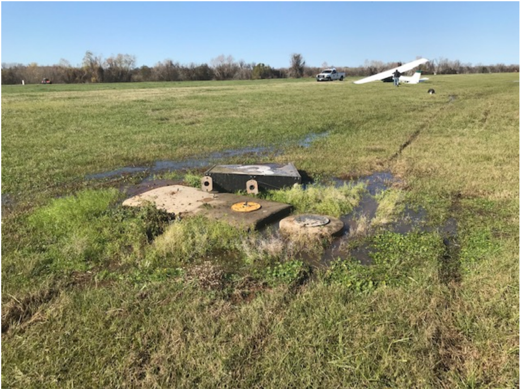
Photo 1 – View of damaged airport sign (Photo courtesy of the FAA)
