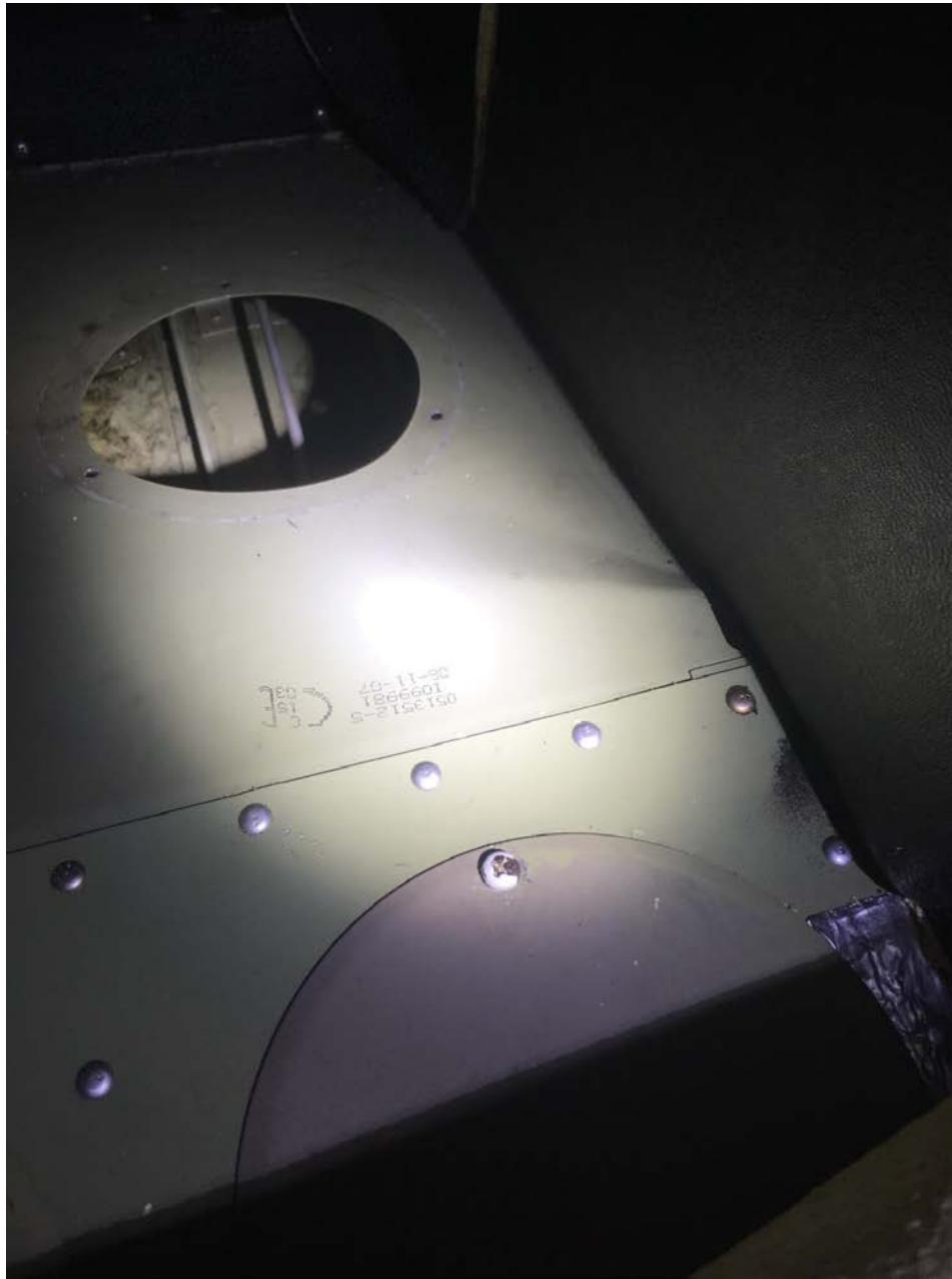
Photo 1 – View of damaged floorboards (Photo courtesy of the FAA)
