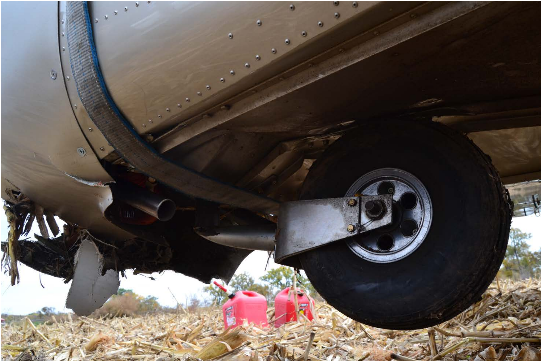
Photo 2 – View of damage to the lower fuselage longerons (Courtesy of FAA)
