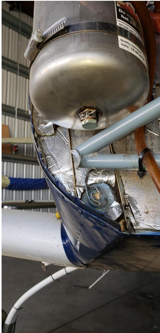
Photo 1 – View of damaged lower right engine mount (Photo courtesy of the FAA)
