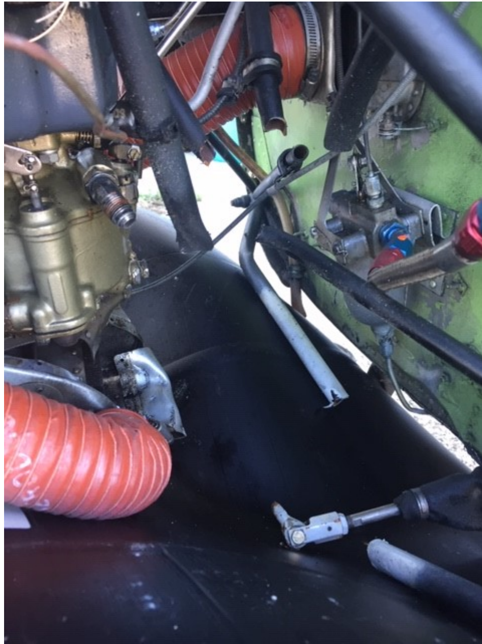
Photo 2 – View of engine frame damage (courtesy of the FAA)
